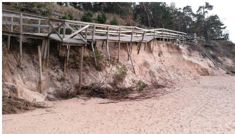
Figure 1. Storm caused erosion of the White Dune slope in October 2018. Inčupe riverbed was filled with sand and retreated from the slope.
